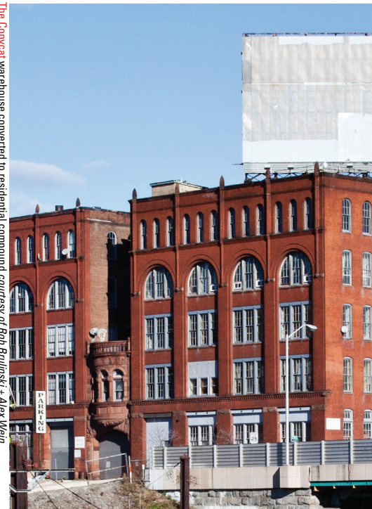
The Copycat warehouse converted to residential compound courtesy of Rob Brulinski + Alex Wein
